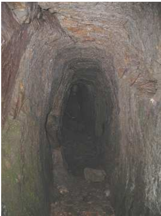
Blick in den Stollen
